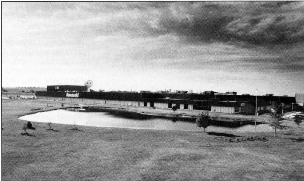
The expansive Kawasaki Motors Manufacturing (KMM) plant in Lincoln, Neb.
