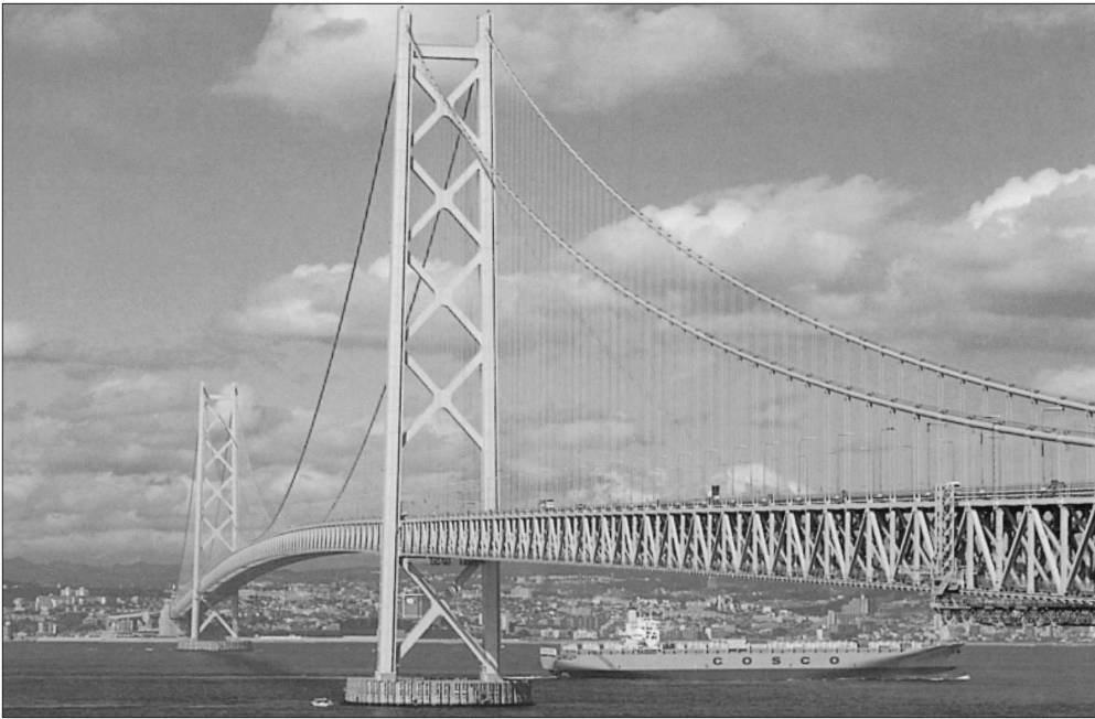
Akashi Kaikyo Bridge in Kobe Japan.
